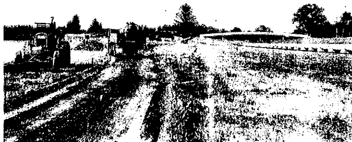
Cyclist-pedestrian path under construction.
