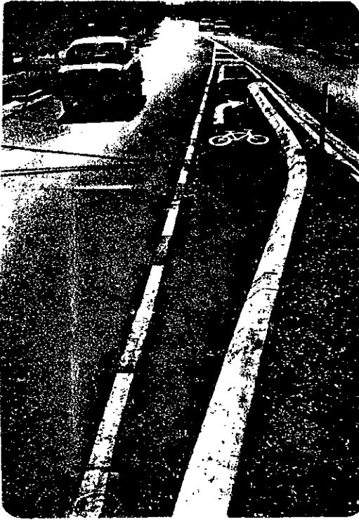
6. Exclusive cyclist only right-hand turn and cut out through median to give access from East Avenue into Cromer Parade.
